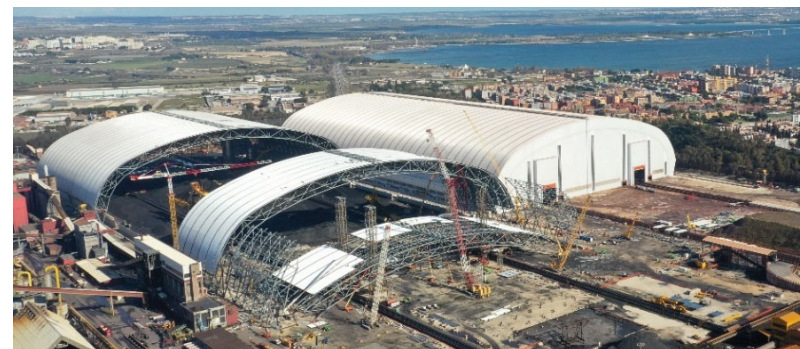
Taranto Feb 20: LHS ongoing Coal yard where we are also erecting the new stacker reclaimers; RHS is finished iron ore yard
