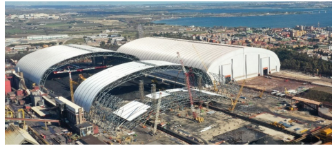
Taranto Feb 20: LHS ongoing Coal yard where we are also erecting the new stacker reclaimers; RHS is finished iron ore yard
